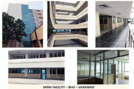
SATHI FACILITY – BHU – VARANASI
