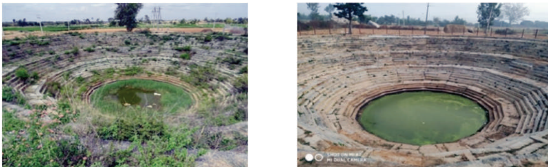
Fig. Kalyani in Rangasthala, Chikkaballapura taluk before and after rejuvenation
